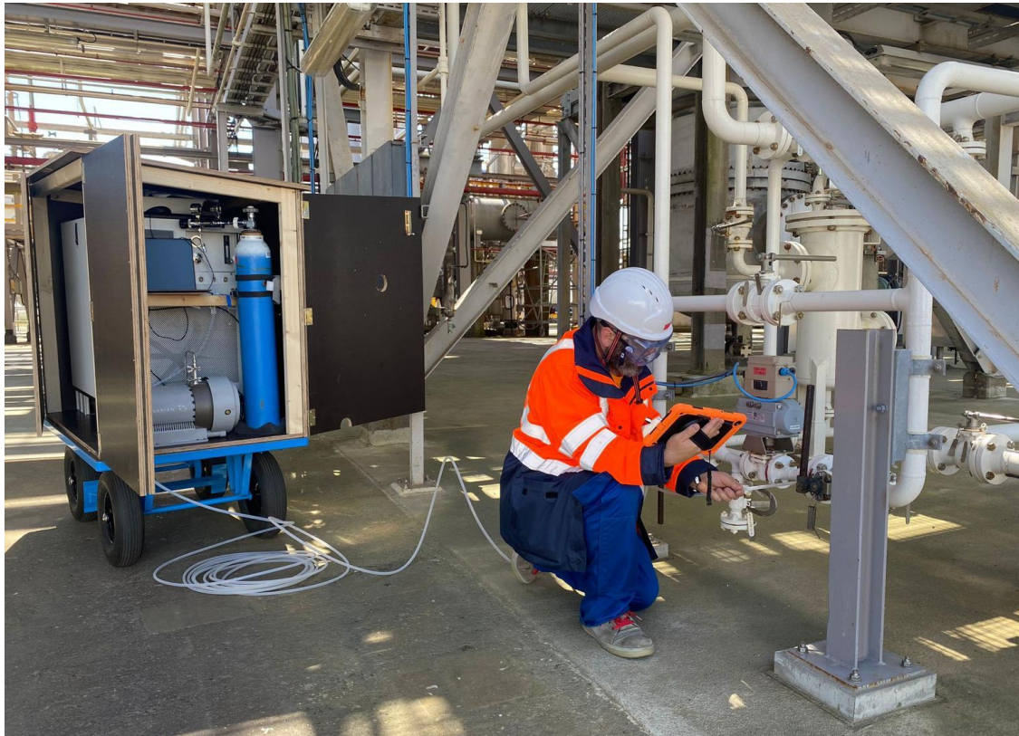
Figure 2: Operator locating the source of an emission using the live data streamed to mobile display. On the left, the simple but effective mobile PTR-TOF platform can be seen.
